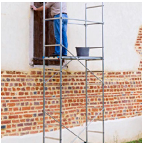
A scaffold tower for a variety of tasks
