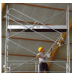
Easy installation of one-piece guardrails
